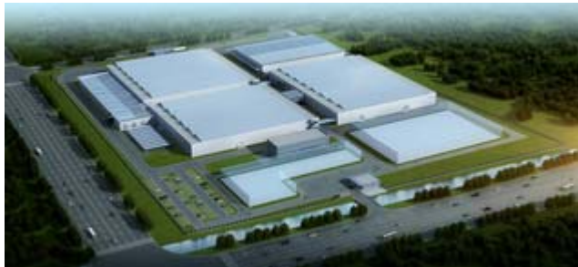
Rieter Changzhou Plant 2 – Overview
