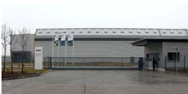
Rieter Changzhou Plant 2 - North Entrance
