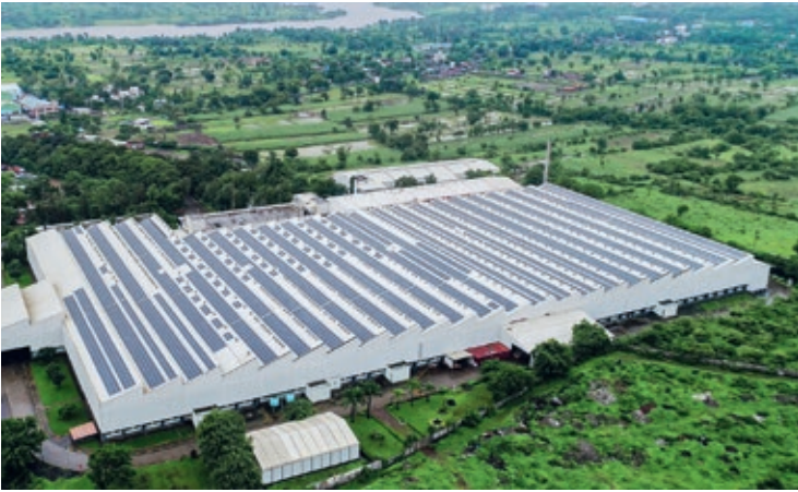
The solar system at Rieter India supplies 25% of the power consumption required annually and reduces CO 2 emissions by 2 500 tons/year.
